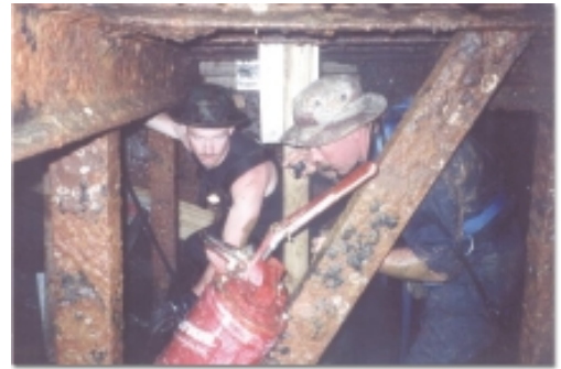
MMC Riendeau and BM2 Ogg install shoring on a damaged bulkhead below the waterline.
