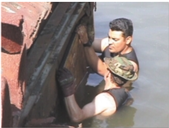
MMC Riendeau and SM2 Guillen install an external patch.
